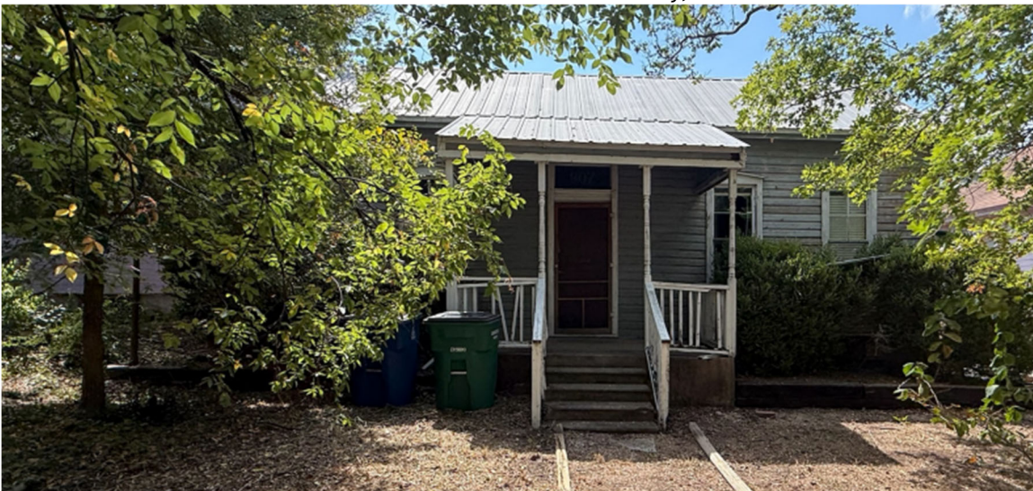
2016 East Austin Historic Resource Survey, HHM Inc.
