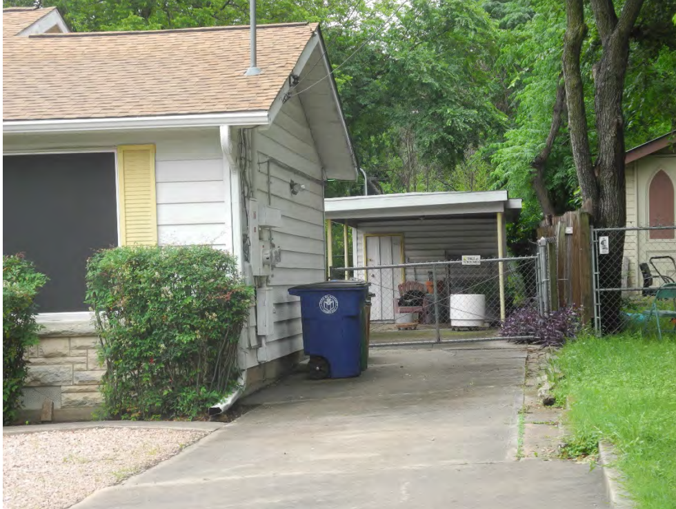
Photo 9: Carport, North & West house facades, camera facing south
