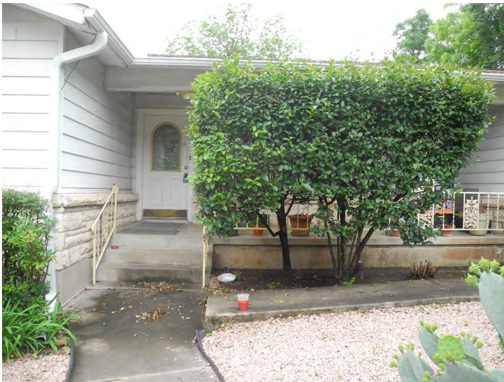
Photo 8: Front Entrance, North façade, camera facing south
