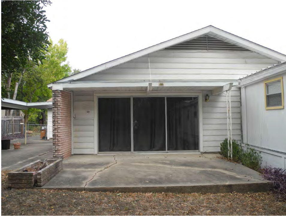
Photo 5: South (rear) façade, camera facing north
