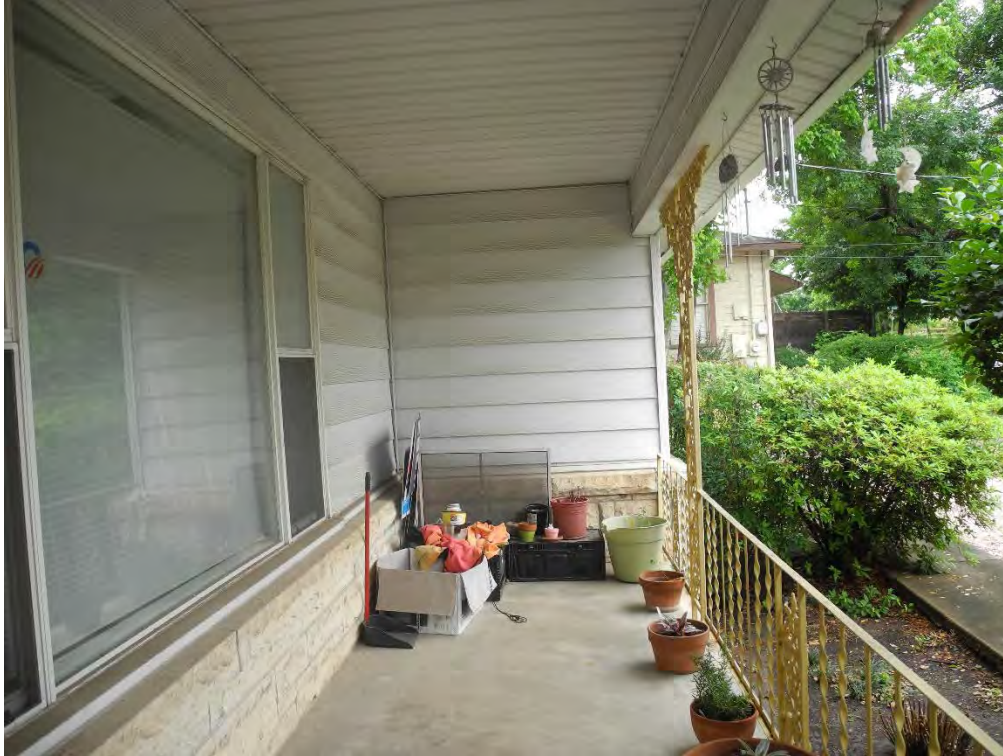
Photo 7: Front porch, North and East Walls, camera facing west
