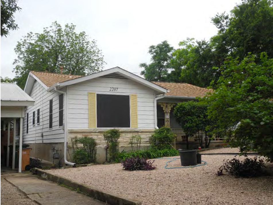
Photo 3: East and North facades, camera facing southwest
