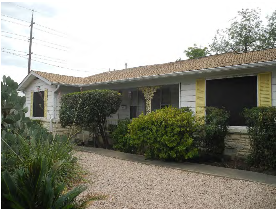
Photo 2: North façade and Inset Porch, camera facing southeast
