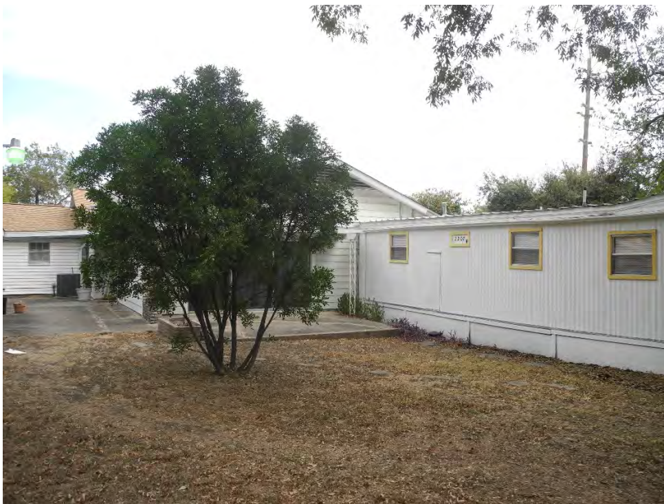
Photo 12: Mobile Home West façade, camera facing northeast
