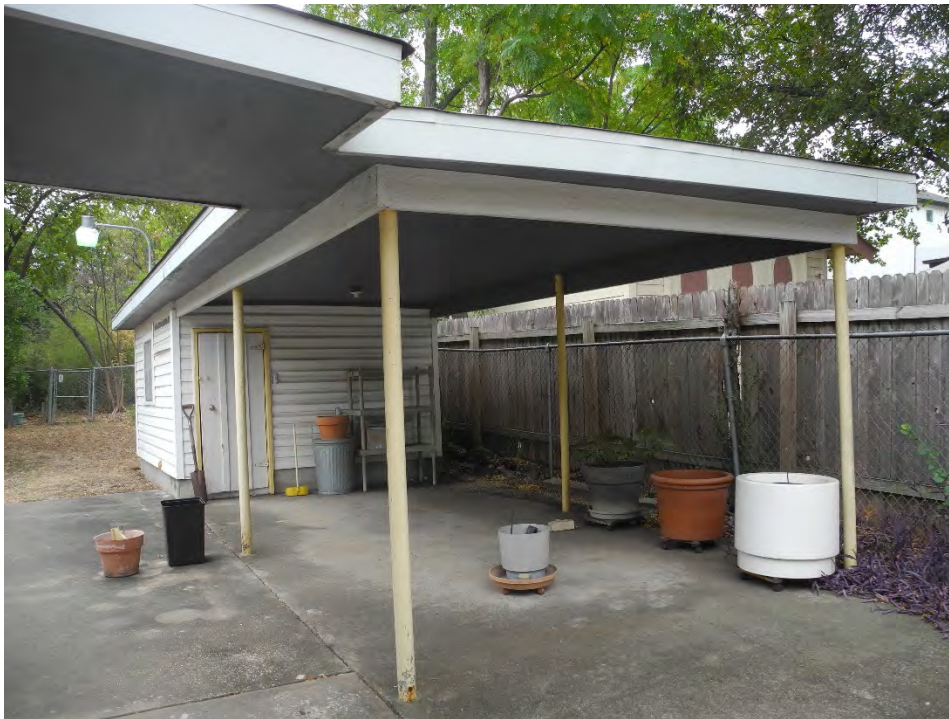
Photo 6: Carport and Shed, East and North facades, camera facing south/southwest
