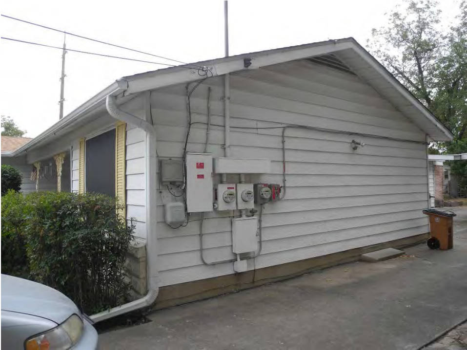
Photo 4: West façade, camera facing southeast
