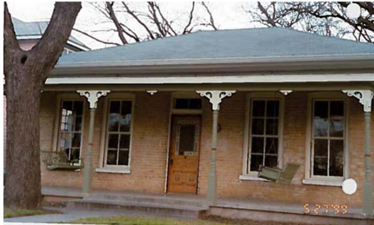
Source: Certificate of Appropriateness for repair, 1999.
