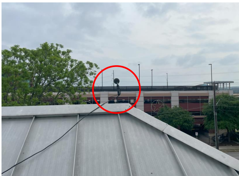
Figure 1. Microphone mounting location on the ridge of the roof of a neighboring property across the street, to evaluate sound transmission level to other properties.
