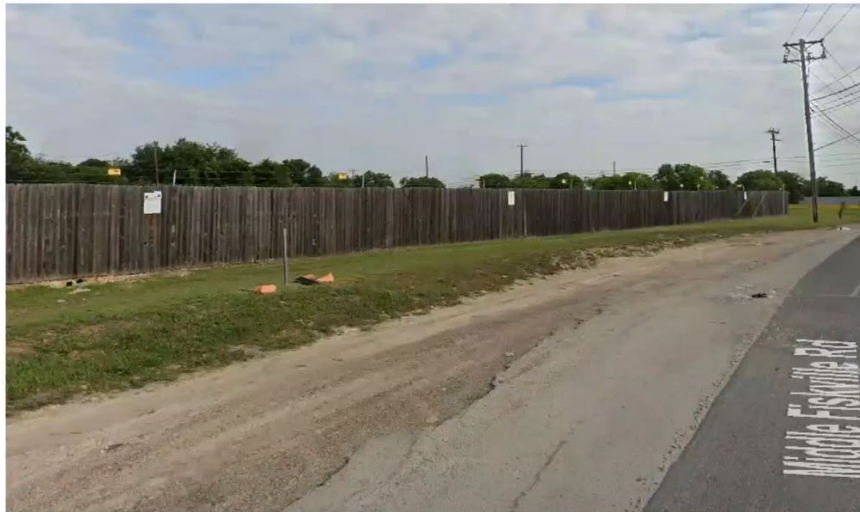
Privacy fence along front of 10602, 10604, 10606, and 10608 Middle Fiskville Road
