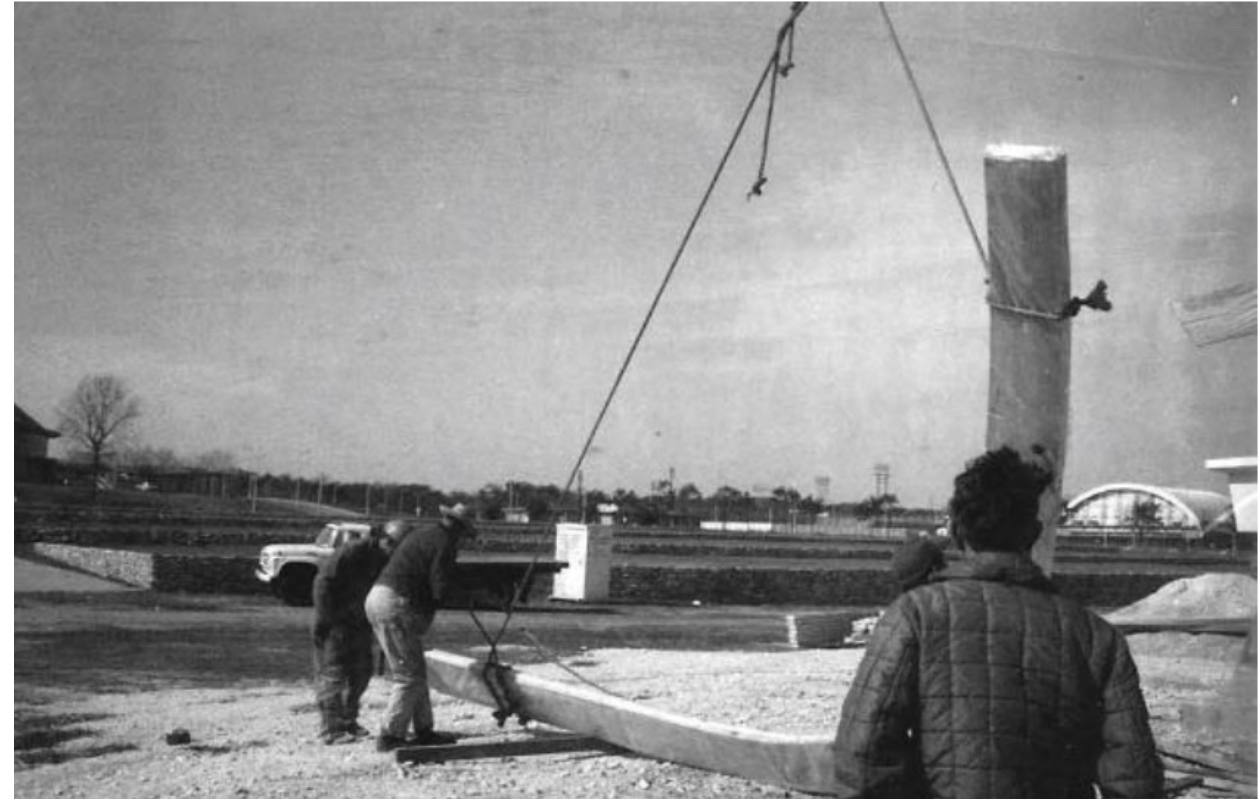
A crane raises one of the glulam beams
