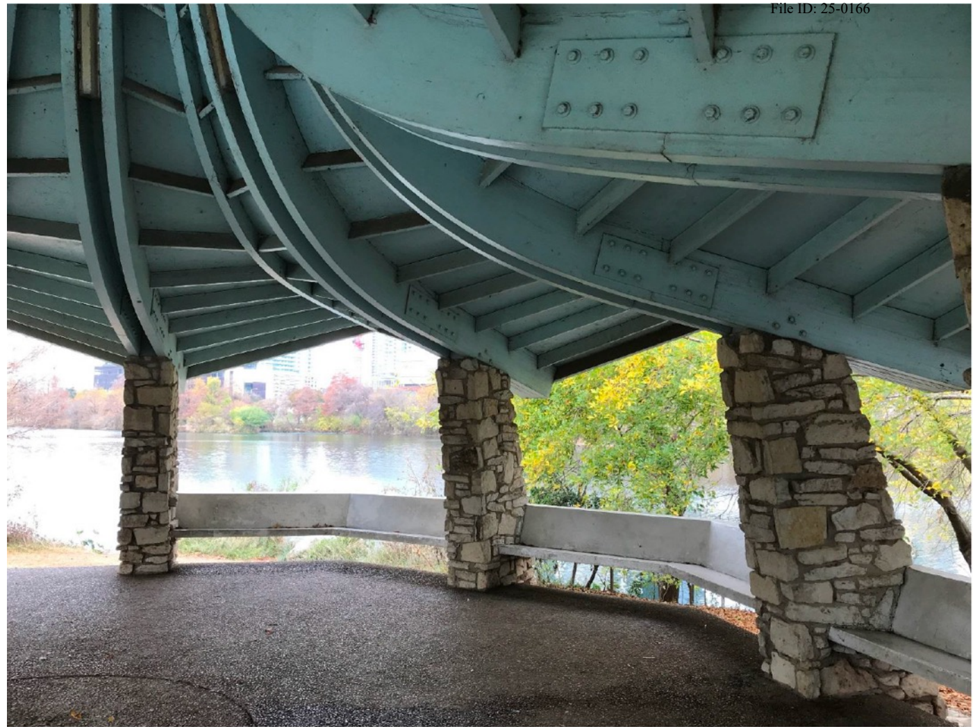
Glulam roof structure
