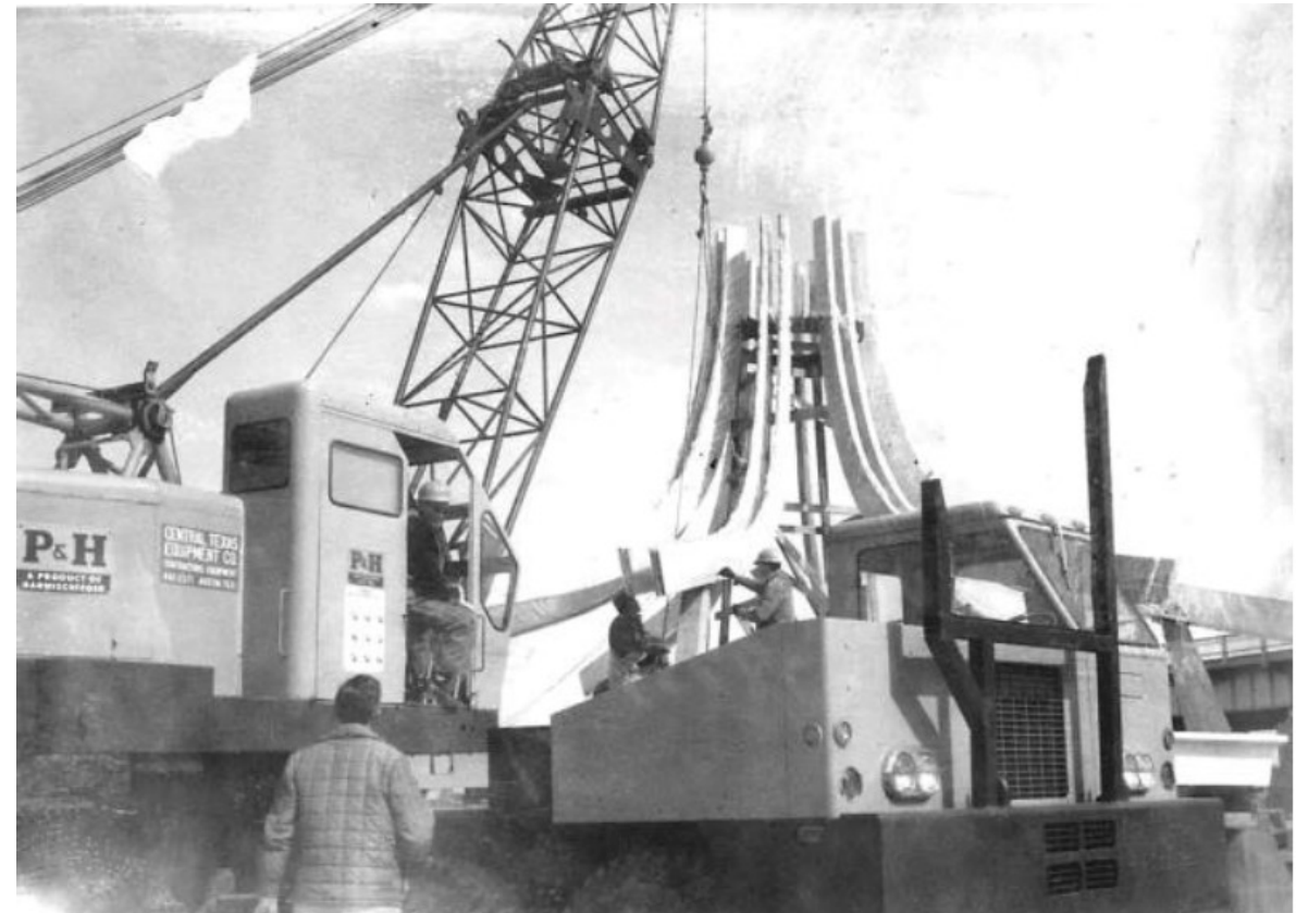
A total of 16 beams support the roof.
