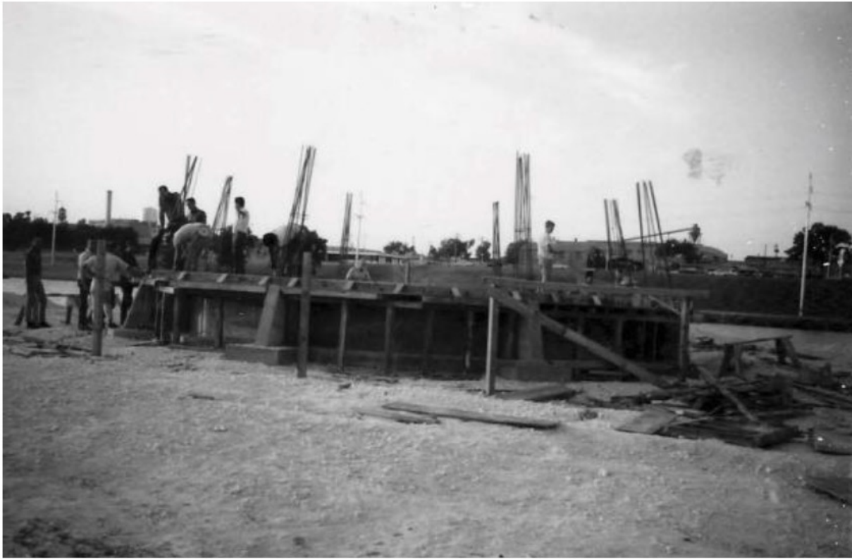
Setting up the formwork for the octagonal slab.
