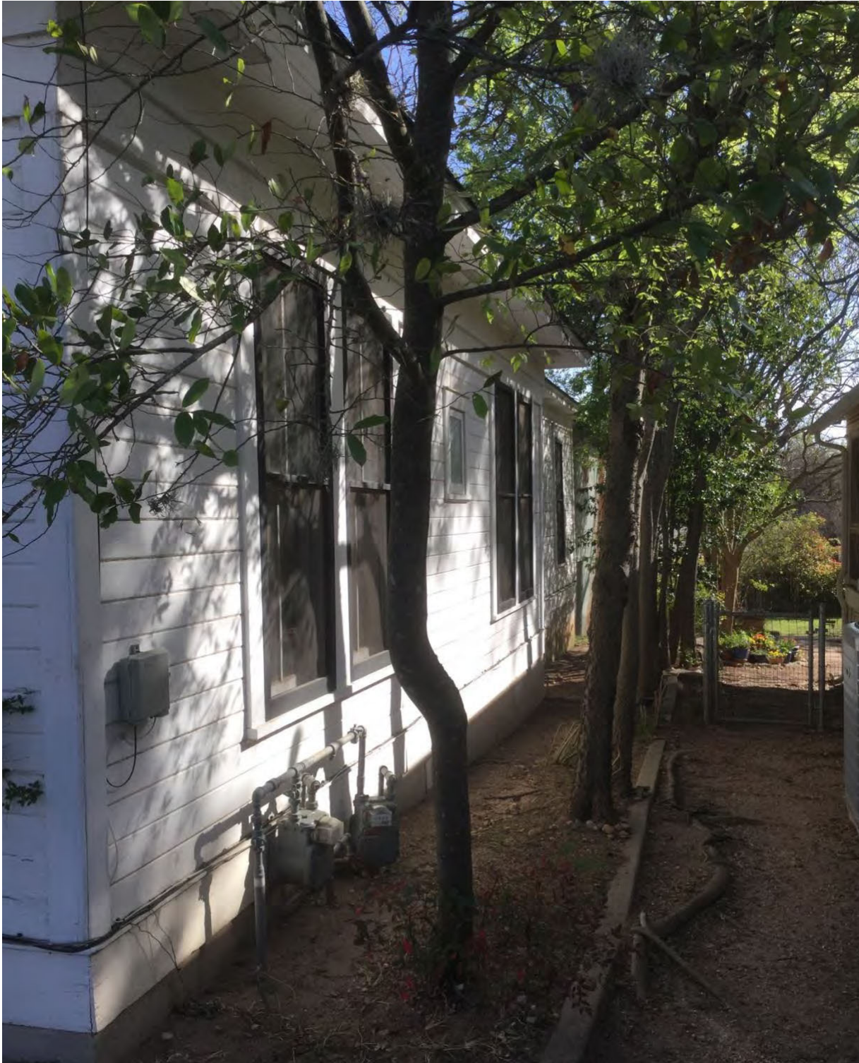
Photo 4 West elevation Camera facing southeast Photo by Tere O'Connell
