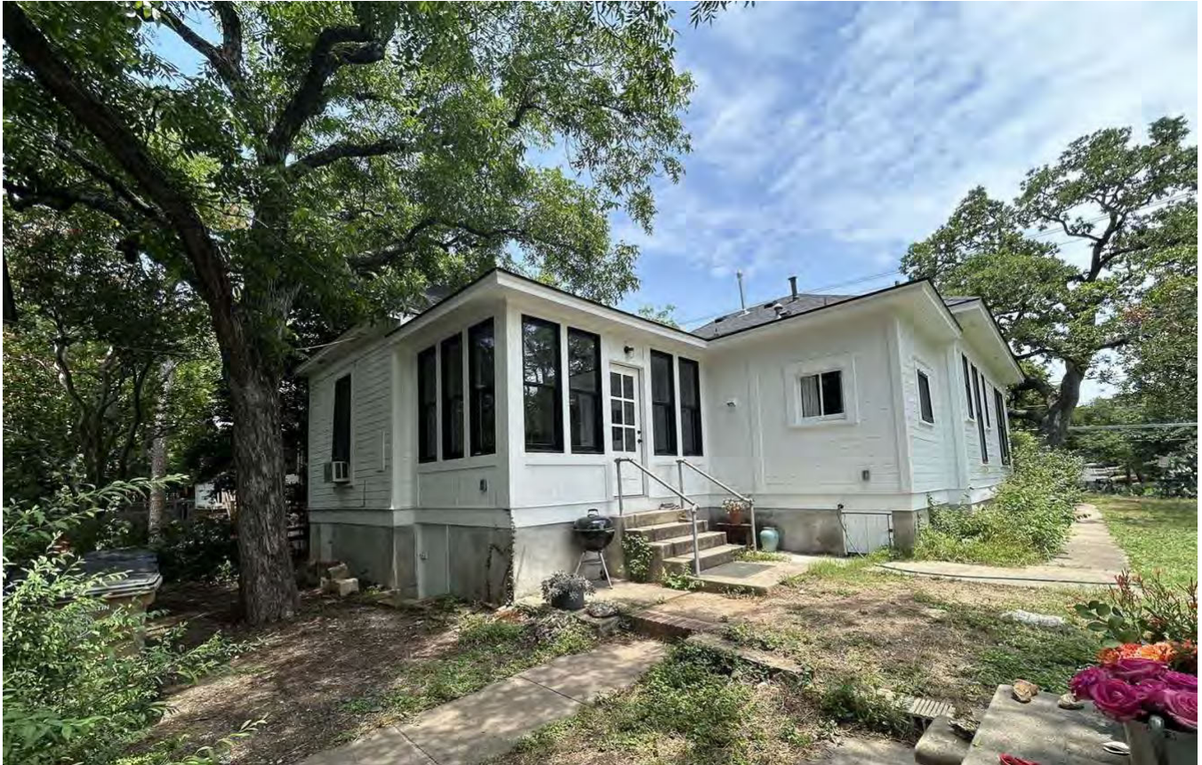
Photo 3 South elevation Camera facing northeast Photo by Lori Martin
