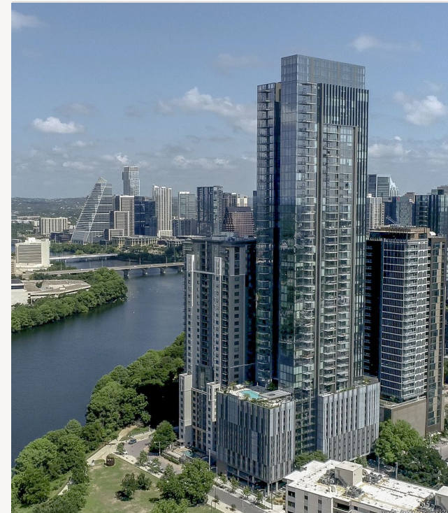
44 East Avenue, 570 ft height
