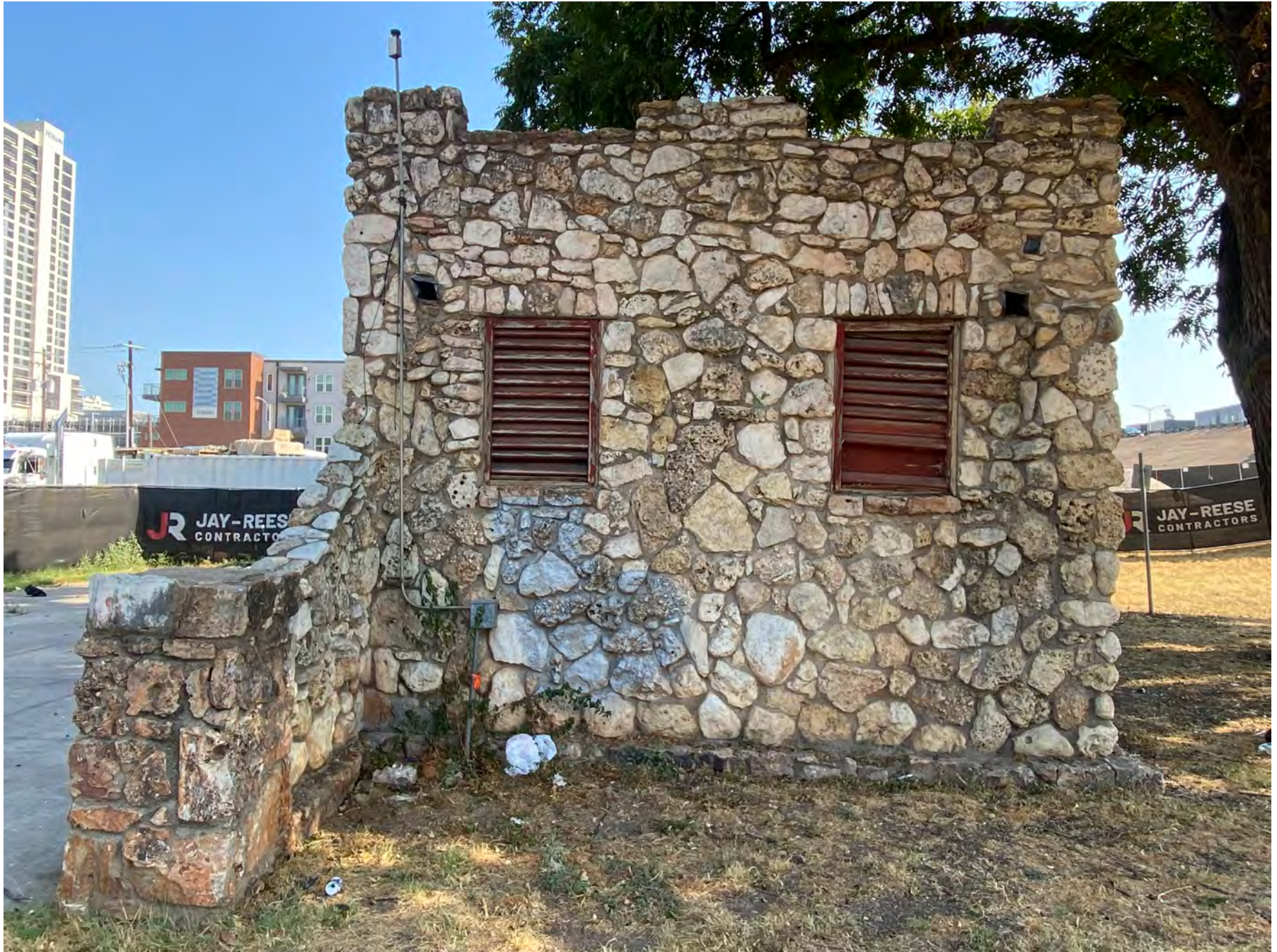
F.5 - HISTORICAL DOCUMENTATION - PHOTOGRAPHS SOUTH ELEVATION. 09/01/2023
