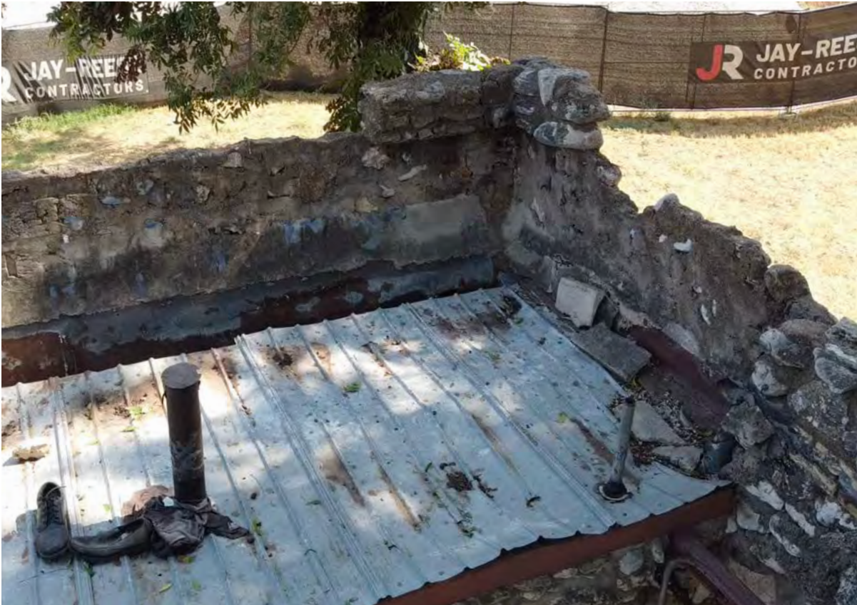
Shelter House Existing Condition
