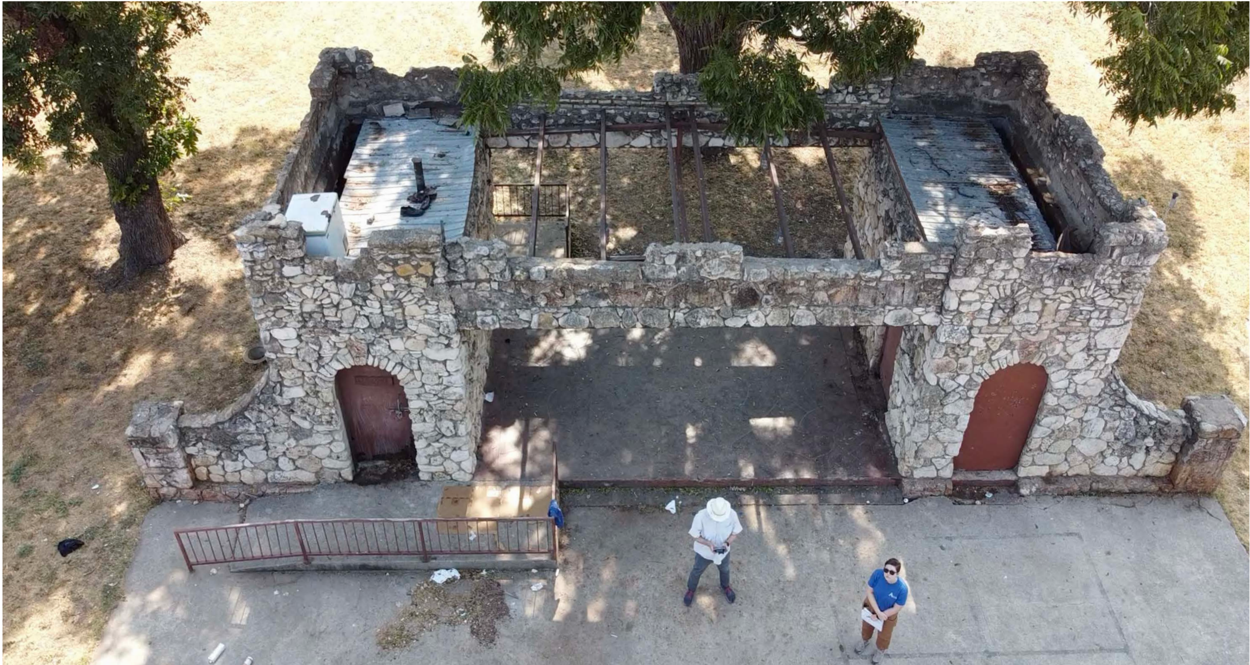
Shelter House Existing Condition
