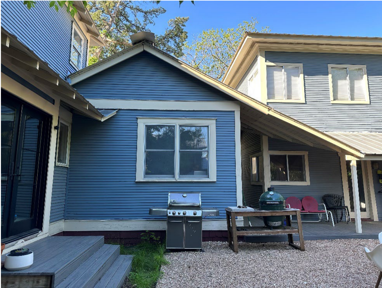
Photo 9. North façade of main building in context with rear addition, camera facing south, 4310 Avenue H. Photo by HHM, April 2024.
