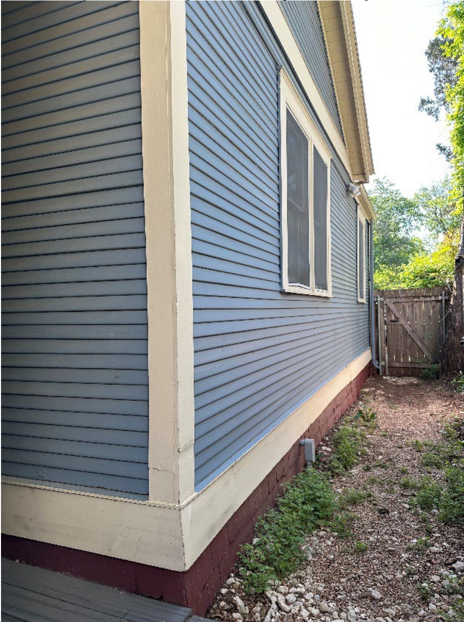
Photo 12. Oblique view of south façade, main building, camera facing northeast, 4310 Avenue H. Photo by HHM April 2024.
