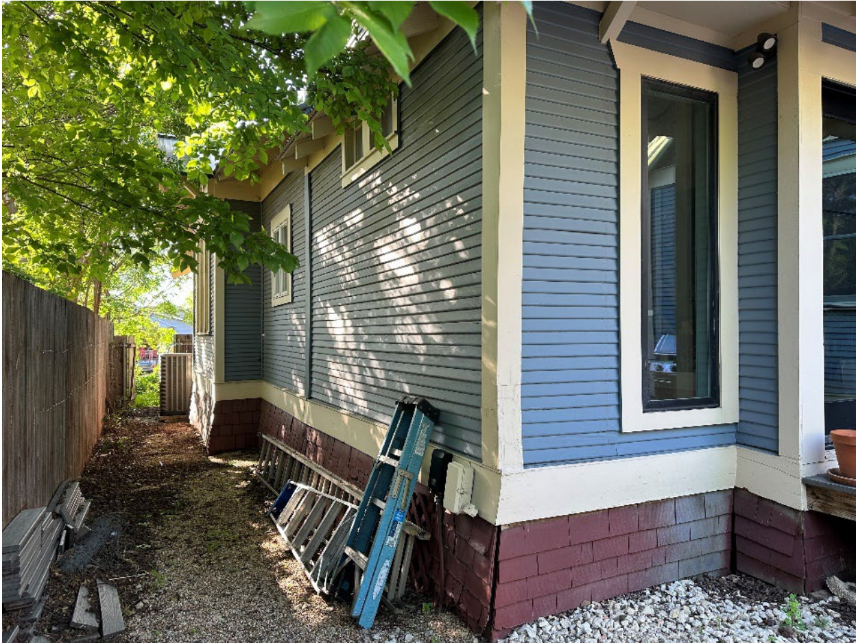
Photo 5. Oblique view of the north side façade, camera facing southeast, 4310 Avenue H. Photo by HHM, April 2024.
