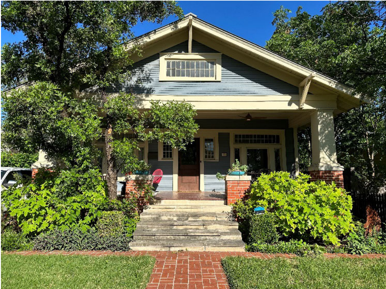
Photo 2. Primary façade, from the end of the front walkway camera facing west, 4310 Avenue H. Photo by HHM, April 2024
