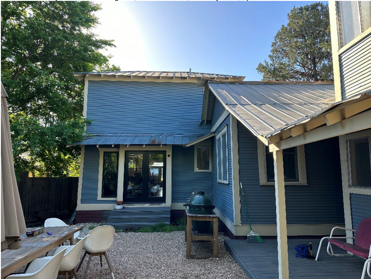
Photo 7. Rear façade, camera facing east, 4310 Avenue H, Photo by HHM, April 2024.
