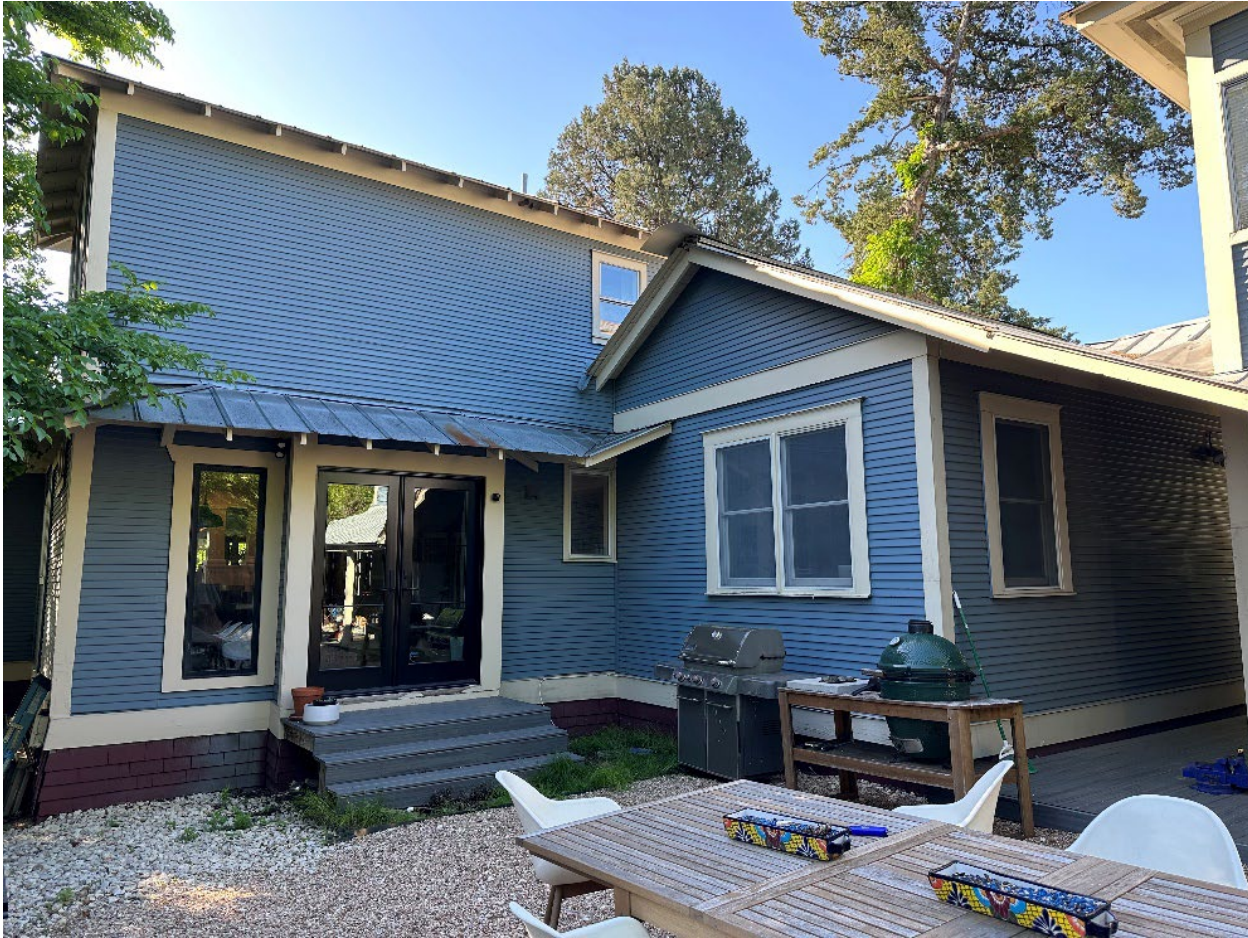
Photo 6. Oblique view of the rear façade, camera facing southeast, 4310 Avenue H, Photo by HHM, April 2024
