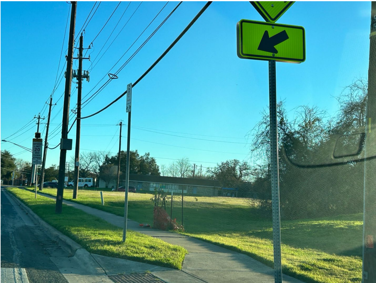
Facing south at 3 rd egress/ingress of 3. Hardly any room between egress/ingress and crosswalk and no parking zone
