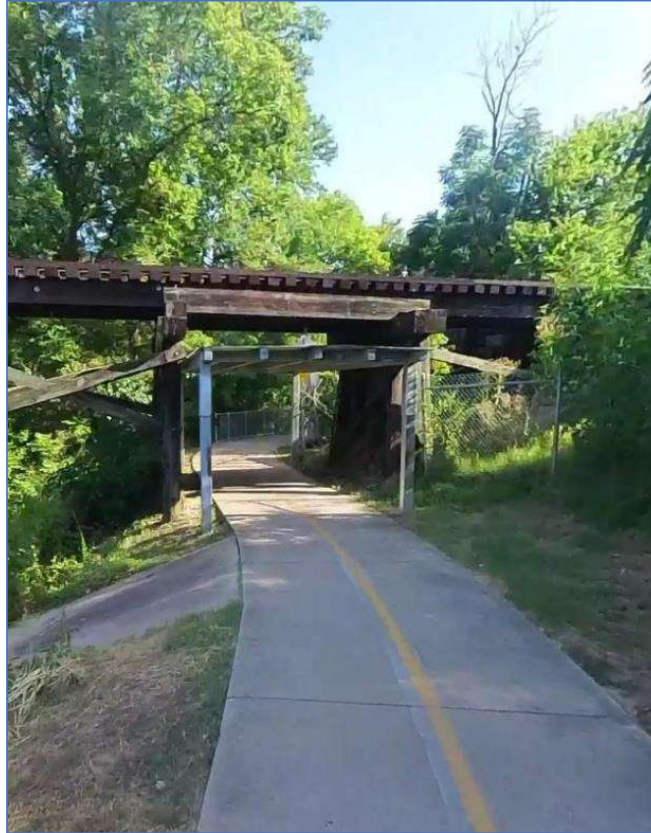
MoKan Rail Crossing at Delwau Lane
