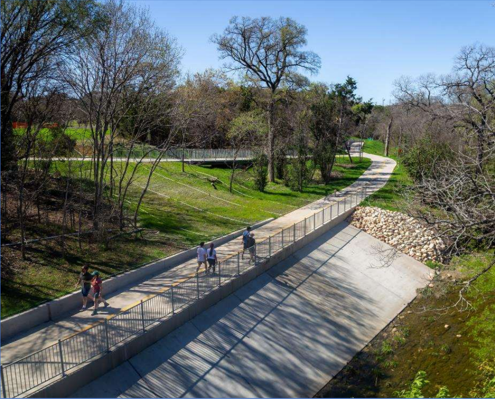
Northern Walnut Creek Trail
