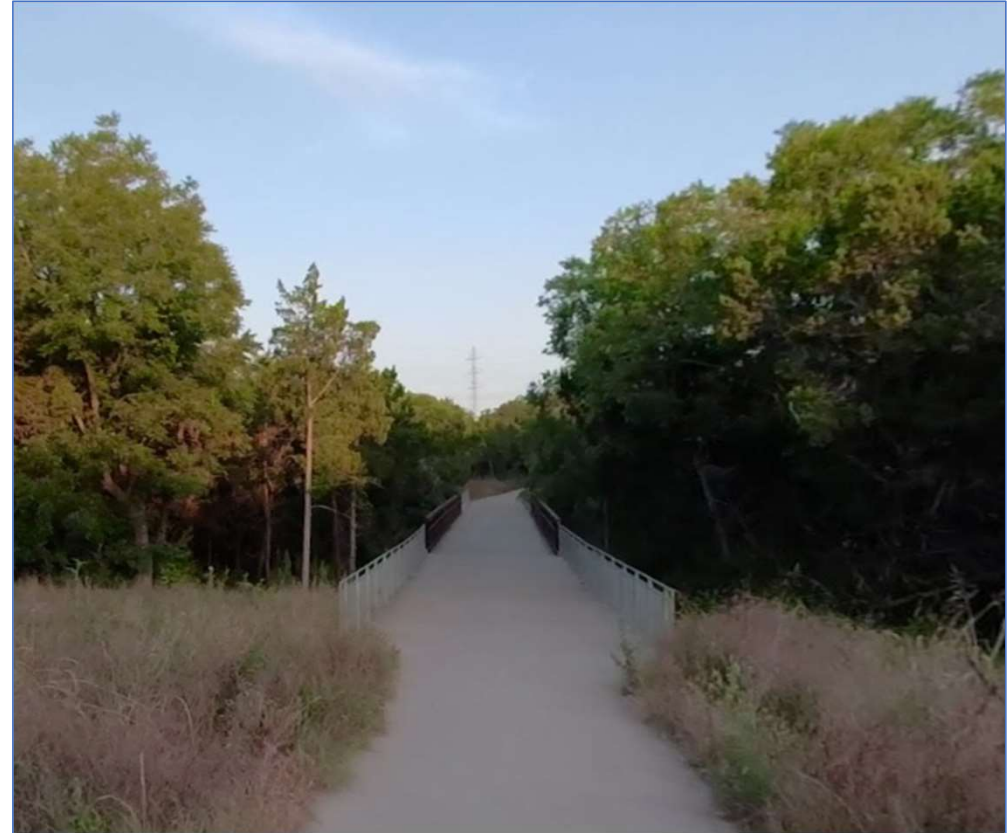
Bridge over Walnut Creek – Walnut Creek Metropolitan Park
