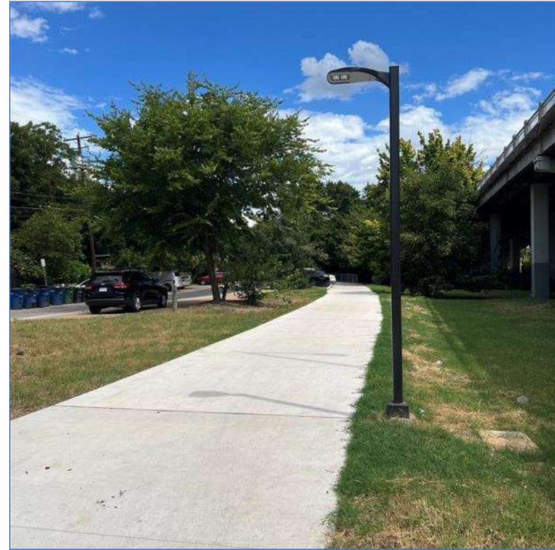
On Gonzales Street heading toward Tillery intersection
