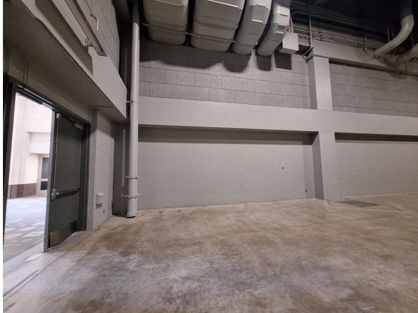
[Riffs and Rhythms Convention Center Mosaic Back CMU of Exhibit Hall 1 Wall 2]
