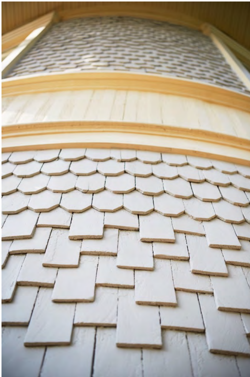
Upper left: Original Corinthian porch capital and column Left: Reinforcement added to turret Upper right: Original fish scale shingles on turret
