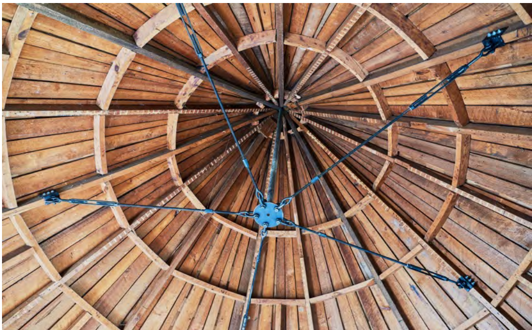
Upper left: Original Corinthian porch capital and column Left: Reinforcement added to turret Upper right: Original fish scale shingles on turret
