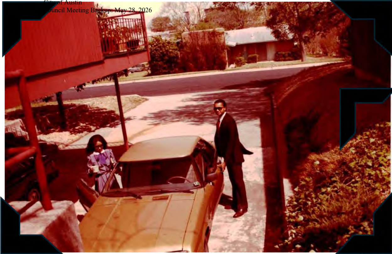
Carport is a defining feature of the house
