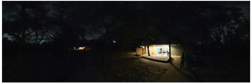
Picture C-157. 360 Image of annex building front entryway
