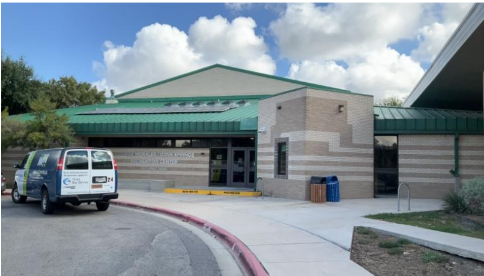
Picture C-60. George Morales Dove Springs Recreation Center - Natural Surveillance
