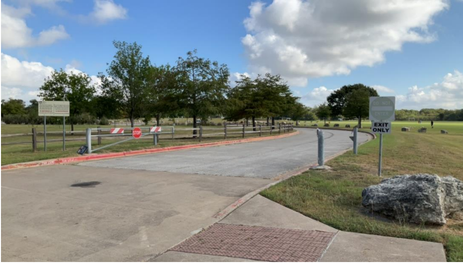
Picture C-51. Onion Creek Soccer Complex - Site / Target Hardening
