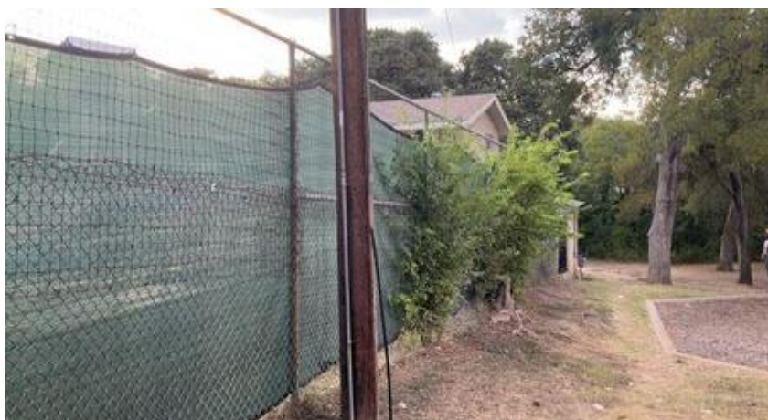
Picture C-71. Big Stacy Pool - Natural Surveillance
