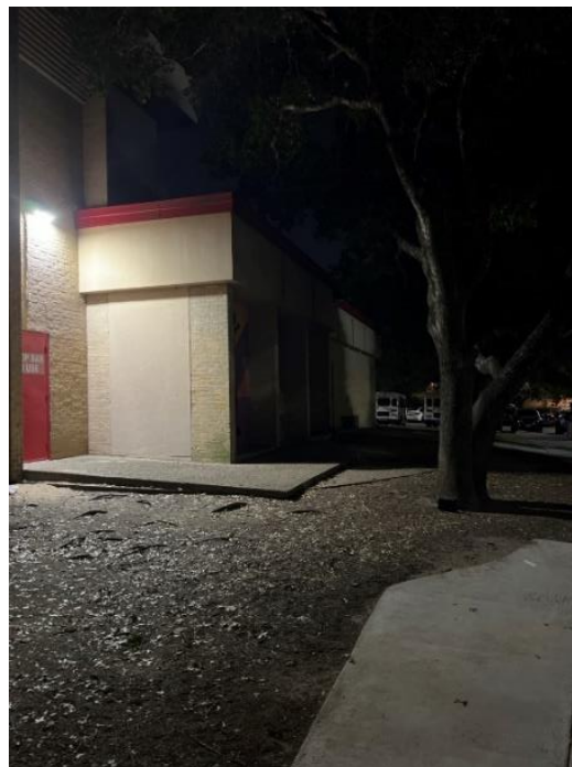
Picture 9. Secondary entry for the South Austin Recreation Center featuring a bright wall-pack and dark corners (taken with phone, no flash)
