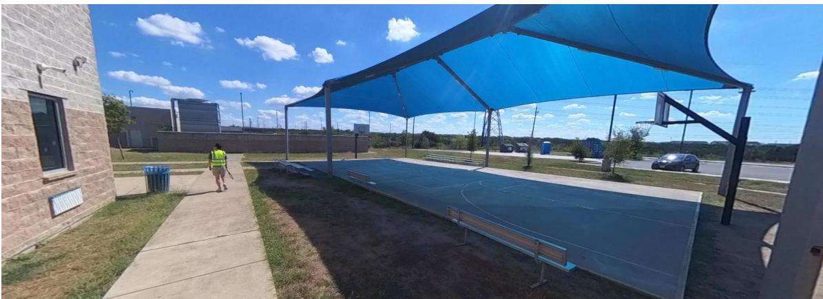
Picture C-48. Turner Roberts Recreation Center - Natural Surveillance
