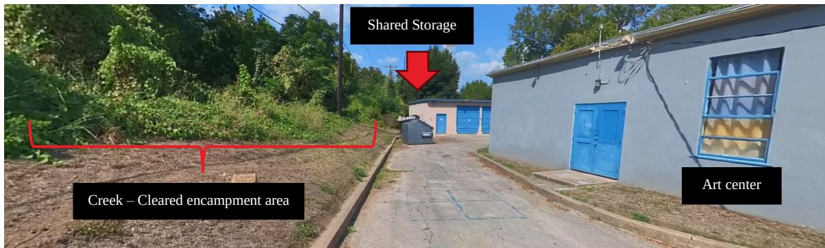
Picture C-45. Dougherty Arts Center - Western side of facility
