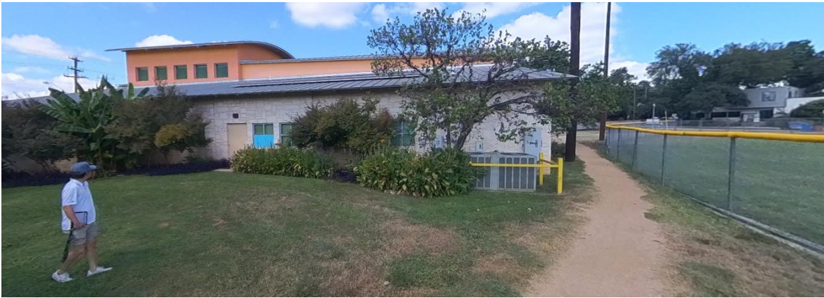
Picture C-58. Lorraine “Grandma” Camacho Recreation Center - Break-in Location
