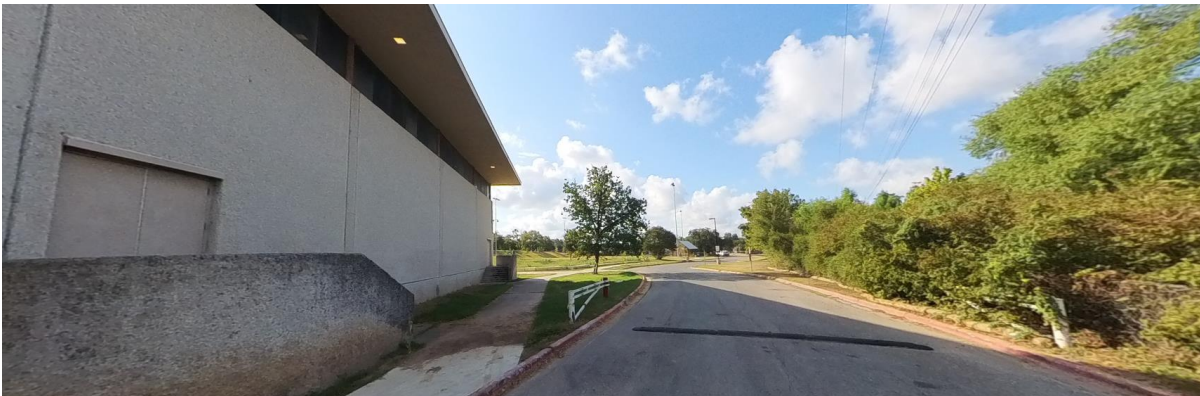
Picture C-82. Givens Recreation Center - Vehicle gates at one side of the district park; the gate on the right has vegetation growing over it, indicating it has not been used in a long time
