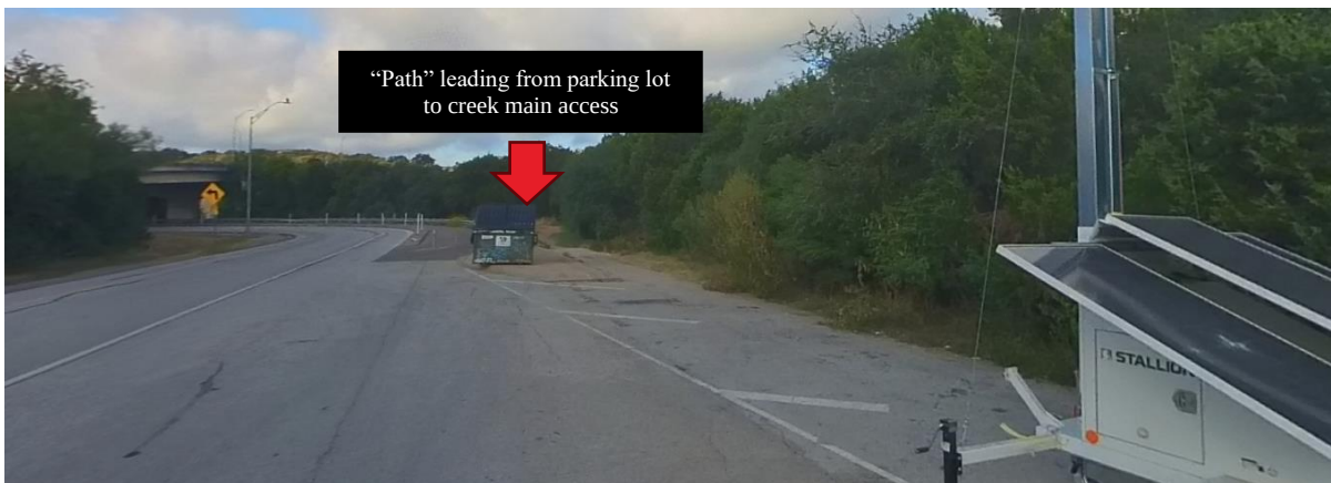
Picture C-33. Barton Creek Wilderness Park - Natural Access Control
