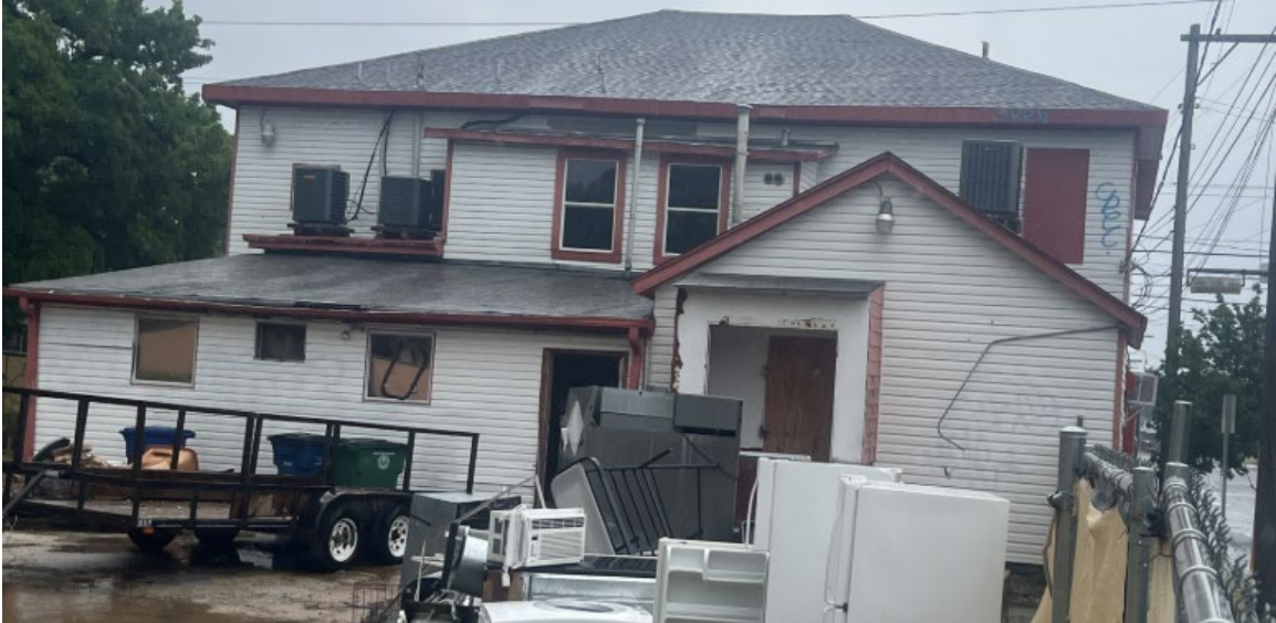
Rear elevation. Source: Demolition permit application, Eureka Holdings, 2024
