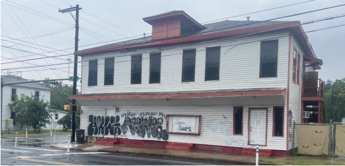
12 th Street (front) elevation. Source: Demolition permit application, Eureka Holdings, 2024
