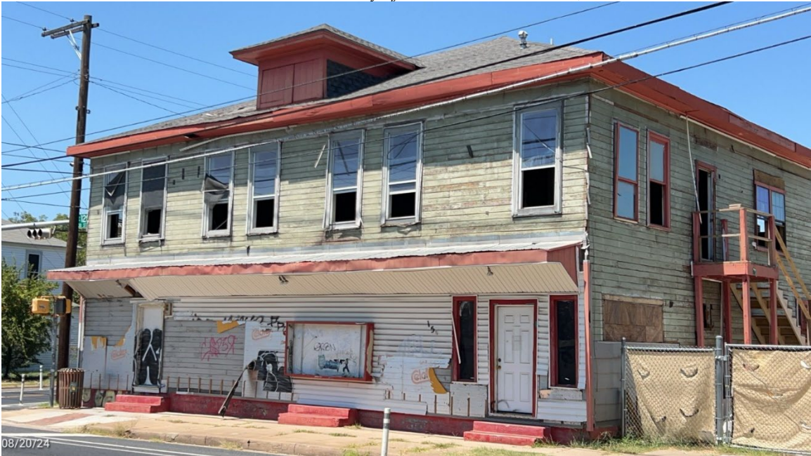
Front elevation. Photo courtesy of Austin Code, August 2024.
