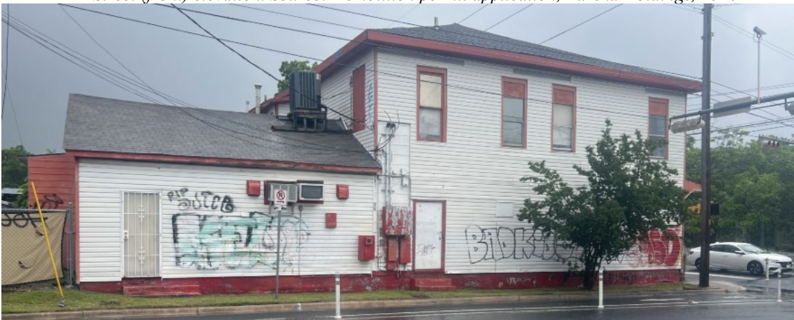
Comal Street (side) elevation. Source: Demolition permit application, Eureka Holdings, 2024
