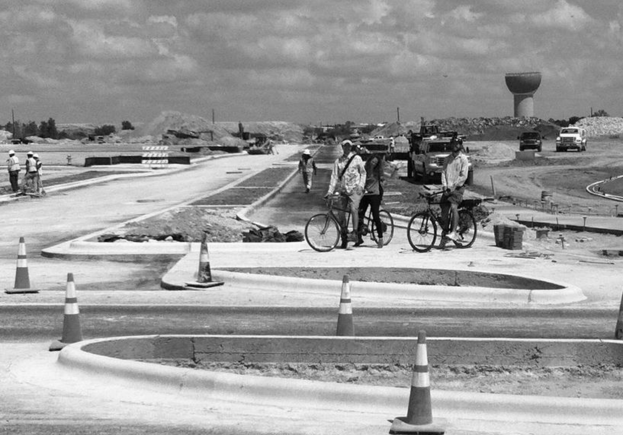
Caption: City bikeway design staff checking on construction of a protected intersection and a planted median separated two-way protected bicycle lanes on Tilley Street in the Mueller Redevelopment.
