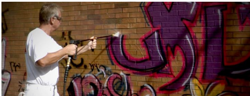
Figure 19. Example of graffiti removal from an exterior surface coated with an anti-graffiti epoxy
