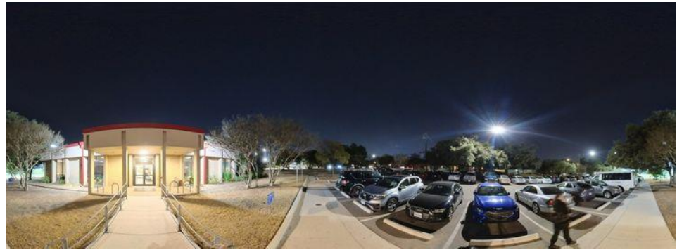
Picture C-150. 360 Image of facility entryway
