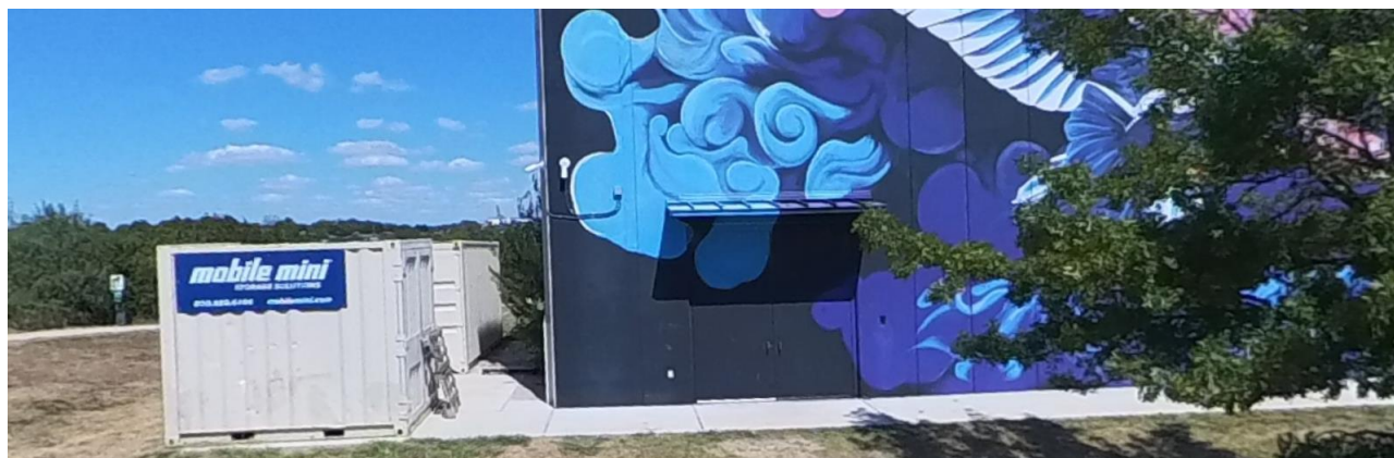
Picture 8. Multiple surveillance cameras are installed at the same building corner and are pointed between and around two shipping containers because of the blind spots they create
