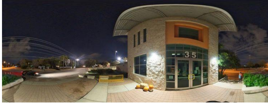
Picture C-166. 360 Image of facility entryway
