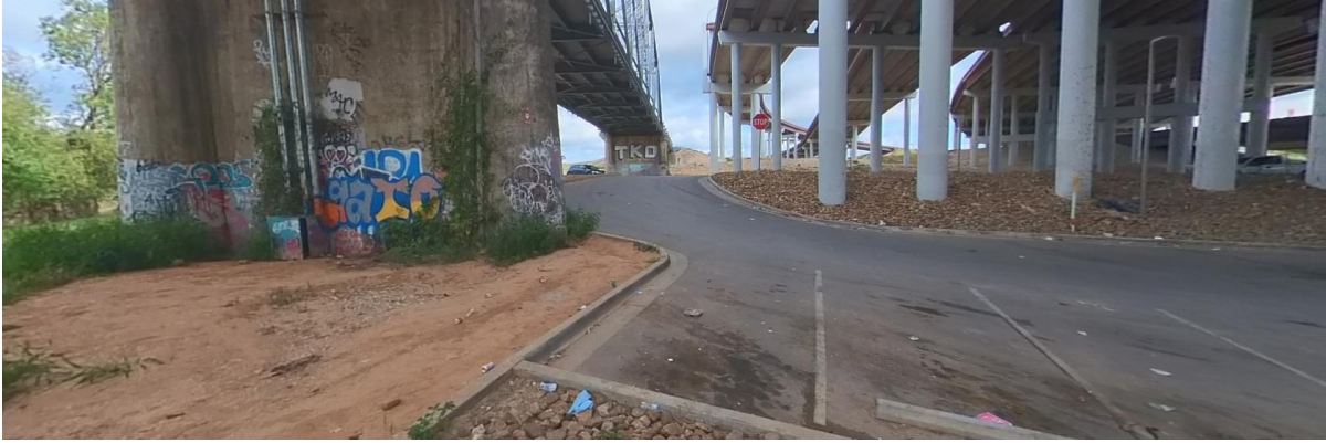
Picture C-38. Colorado River Wildlife Sanctuary - trash littered throughout the parking lot, including extensive graffiti on the pedestrian bridge pillar
