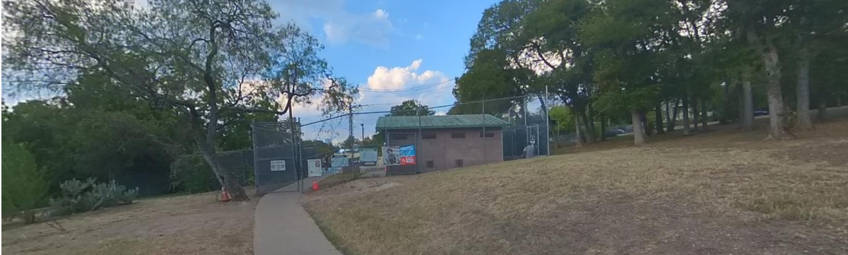
Picture C-72. Big Stacy Pool - Natural Access Control - At the front are the public restroom and shower facility frequently misused by the unhouse population or drug users
