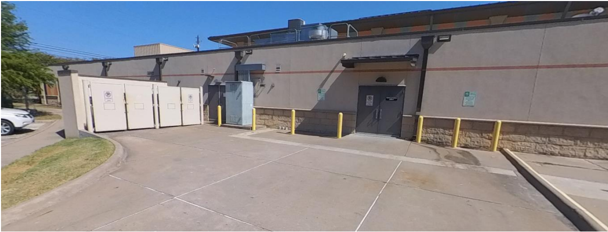
Picture C-47. Asian American Resource Center - Maintenance Area
