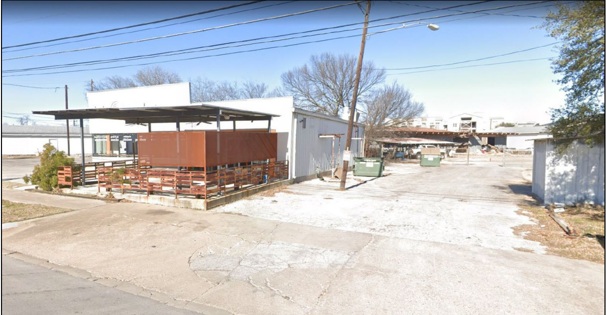
The existing site is developed as several auto-centric office, commercial, and industrial uses.
