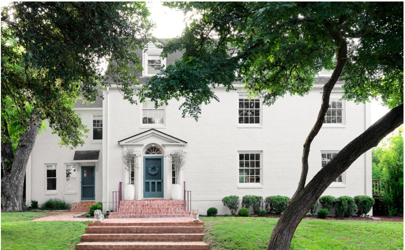
Application photos of exterior viewed from San Gabriel Street
