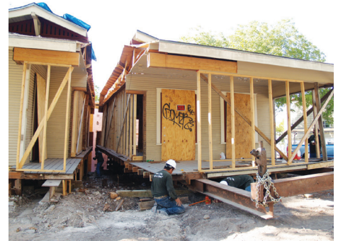
A bungalow is cut and lifted on temporary steel rails in preparation for relocation. (Credits: Ben and Sandi Heimsath)
