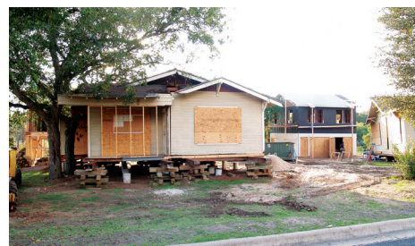
A pair of Duval Avenue bungalows, owned by a University of Texas at Austin fraternity and scheduled for demolition, were sold and relocated to two adjacent lots in the JJ Seabrook Neighborhood. Two 1930s Bergstrom Air Force Base barracks, previously moved to the lots in the 1940s, were also relocated on-site and lifted to become garage apartments. The bungalows and barracks received full renovations, orchestrated and designed by Architect Ben and Sandi Heimsath. (Credits: Ben and Sandi Heimsath)
