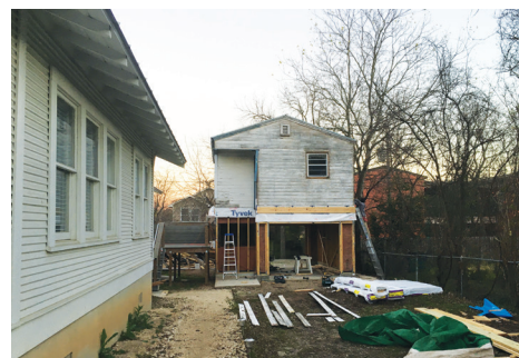
Built in 1937, a garage apartment was lowered, relocated and rotated 180 degrees, then lifted for reuse. In addition to a new exterior stair and one-car garage below, the interior renovation preserved the art deco details, pine flooring, and cabinetry, while adding a new bathroom, HVAC system, and plumbing. (Credits: Sarah Gamble)
