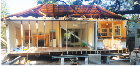
A house is cut in half and temporary wood supports installed to prepare for relocation. (Credit: Kathy Robinson)
