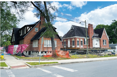
Contributing to a local historic district, two Tudor Revival houses on opposite sides of a block in Gainesville, Florida were relocated to make way for a new sorority house near the University of Florida. Temporary steel rails were inserted through the skirt to lift and support the hybrid structures with their brick façades and wood-framed interiors. (Credits: Carly Walker, Sarah Gamble)
