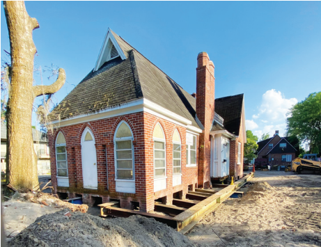
A Tarrytown house (above) is cut into multiple chunks (below) in preparation for relocation. (Credits: Kathy Robinson)
