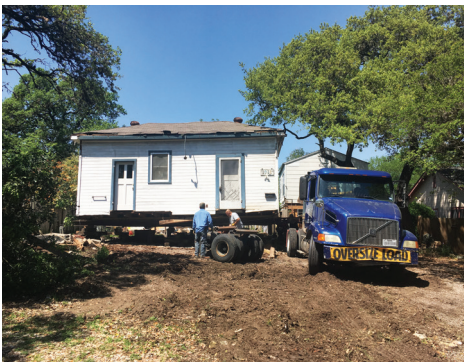
A 1933 main house approved for demolition was purchased by a general contractor and relocated outside of Austin. The porch, which extends the entire length of the front facade, was temporarily removed for transport. (Credit: Sarah Gamble)
