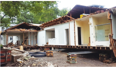
A Tarrytown house (above) is cut into multiple chunks (below) in preparation for relocation. (Credits: Kathy Robinson)
