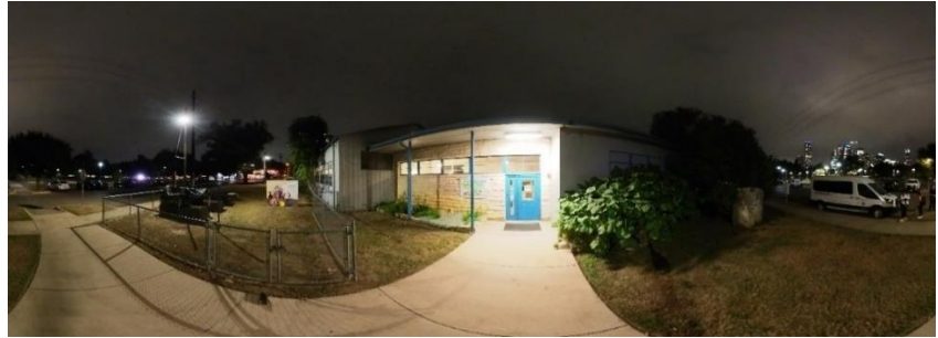
Picture C-141. 360 Image of east entry
