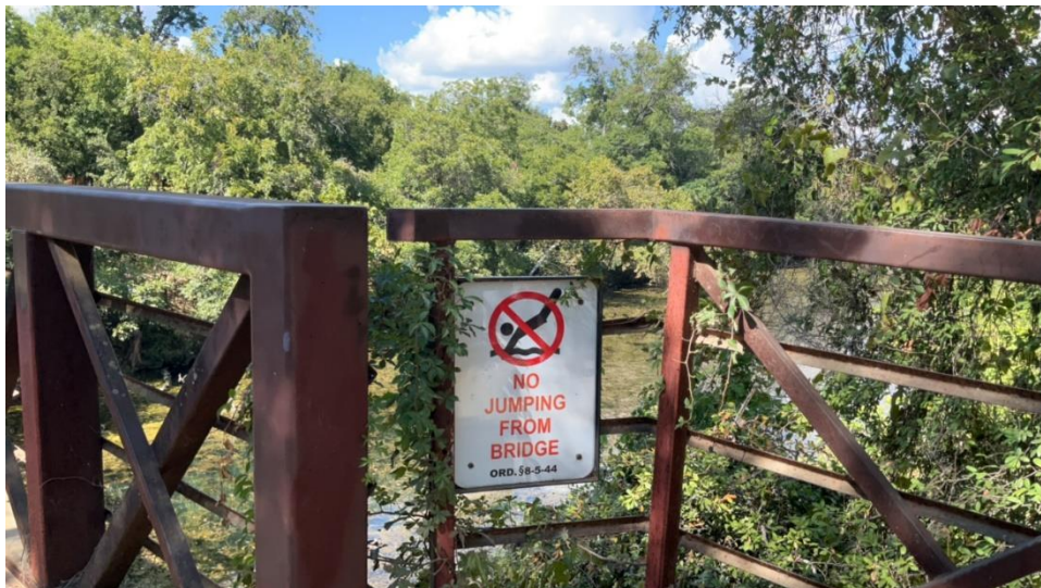
Picture C-12. Zilker Metropolitan Park (Park Center, North) - Image Management / Maintenance
