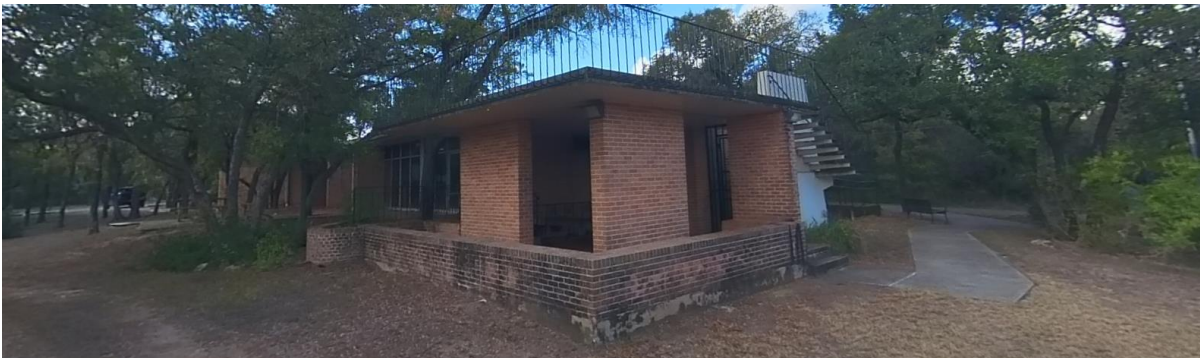
Picture C-70. Danny G. McBeth Recreation Center - The back of the annex building experiences a high number of unknown individuals seeking shelter, using the outdoor power outlet, or consuming alcohol or using drugs
