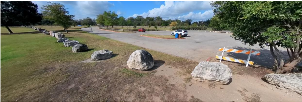
Picture C-52. Onion Creek Soccer Complex - Site / Target Hardening
