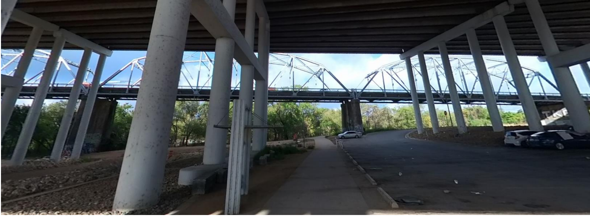
Picture C-36. Colorado River Wildlife Sanctuary - pedestrian bridge adjacent to the greenbelt parking lot which is underneath a major highway
