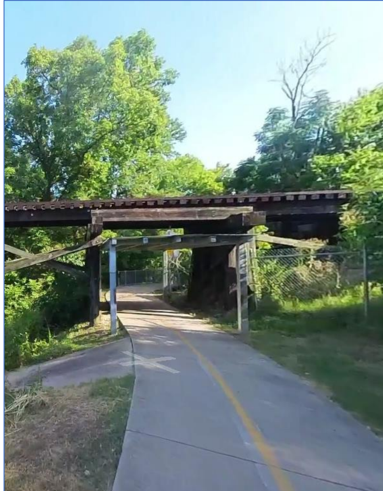
MoKan Rail Crossing at Delwau Lane
