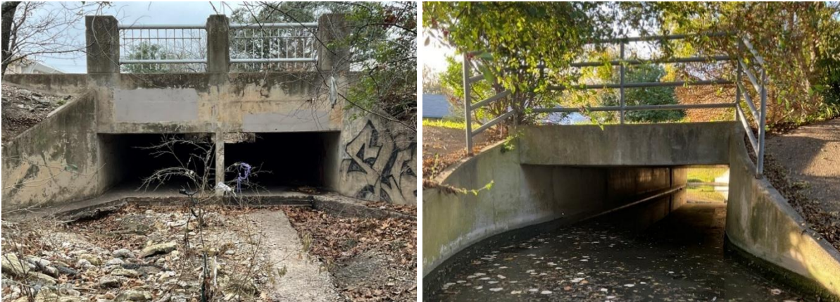
Figure 3. Small Bridge Examples – Box Culverts
