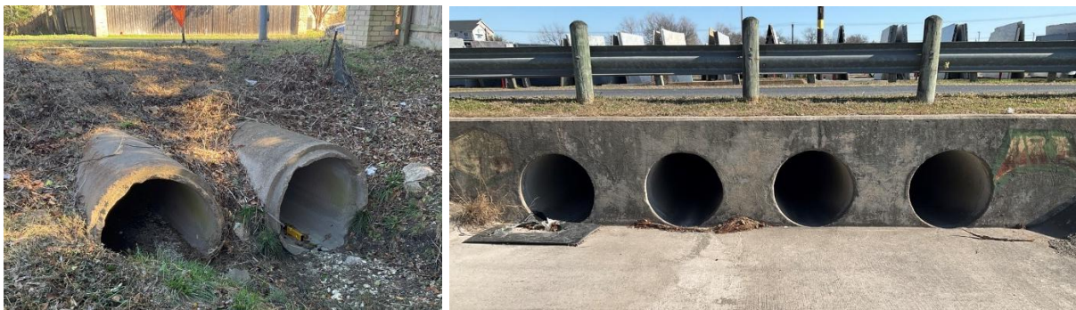
Figure 4. Small Bridge Examples – Pipe Culverts
