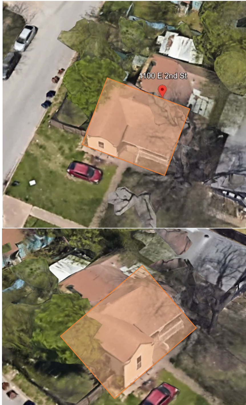
Google Earth images showing intact portion of house constructed during the period of significance ending in 1938. Proposed H zoning will be applied to this portion of the property only.
