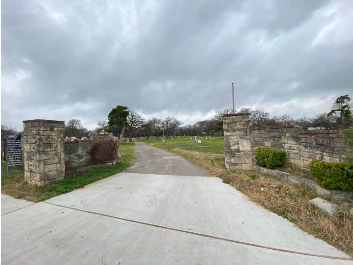
Photo 1. Bethany Cemetery entrance gate, facing southwest from Springdale Road. Photo by Emily Payne, 2025.
