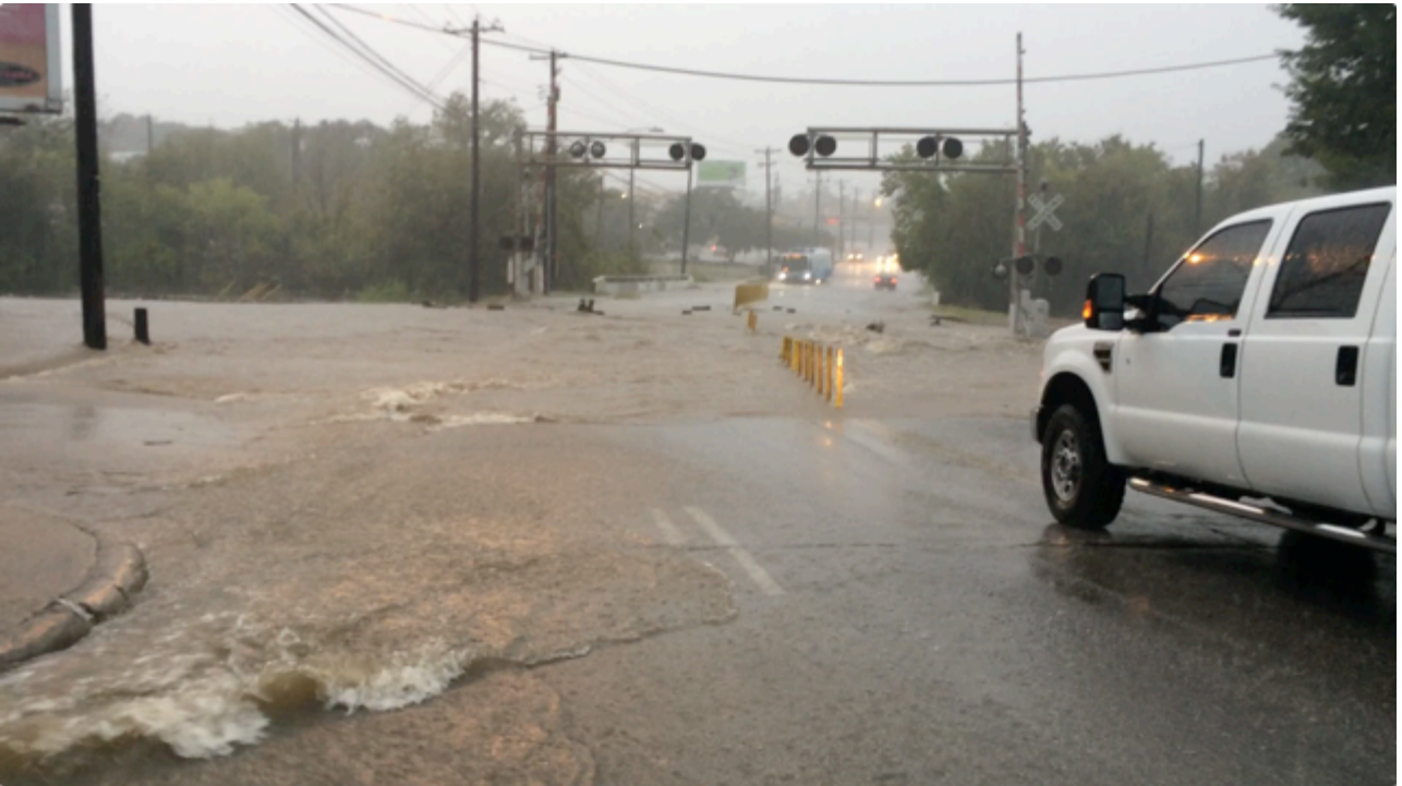
Figure 8 Oltorf Flooding 10-30-15 Photo Courtesy of Peter Williams
