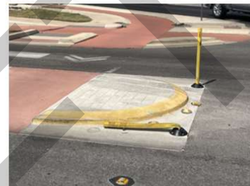
Flattened delineator post
