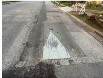
Uneven asphalt speed cushion with missing raised pavement markers (RPMs)
