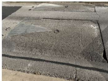
Uneven asphalt speed cushion with missing RPMs
