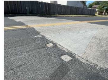
Worn asphalt speed cushion with missing RPMs
