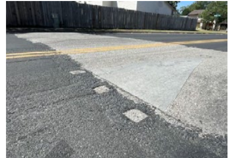
Worn asphalt speed cushion with missing RPMs
