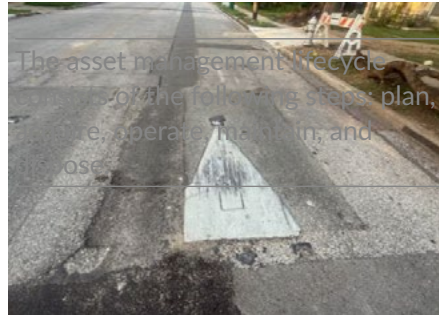
Uneven asphalt speed cushion with missing raised pavement markers (RPMs)
