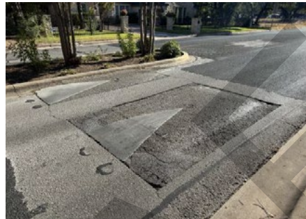
Uneven asphalt speed cushion with missing RPMs
