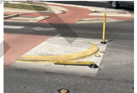
Flattened delineator post
