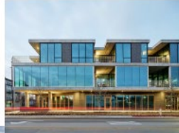
Waterstreet Lofts Residential Cesar Chavez and Comal ~40 feet, above ground parking
